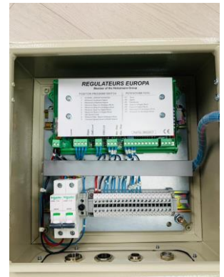
New 1115 Governor Control Card Mounted in Control Panel
