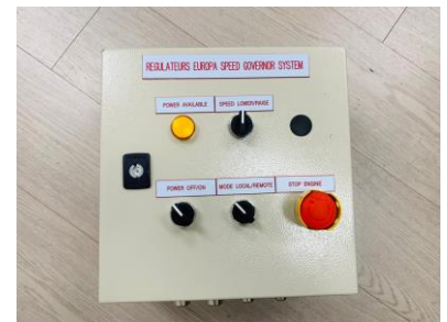
Customised Control Panel with Operative Switches and Tags
