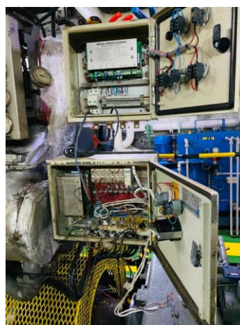
Installation and Wiring of New Control Panel
